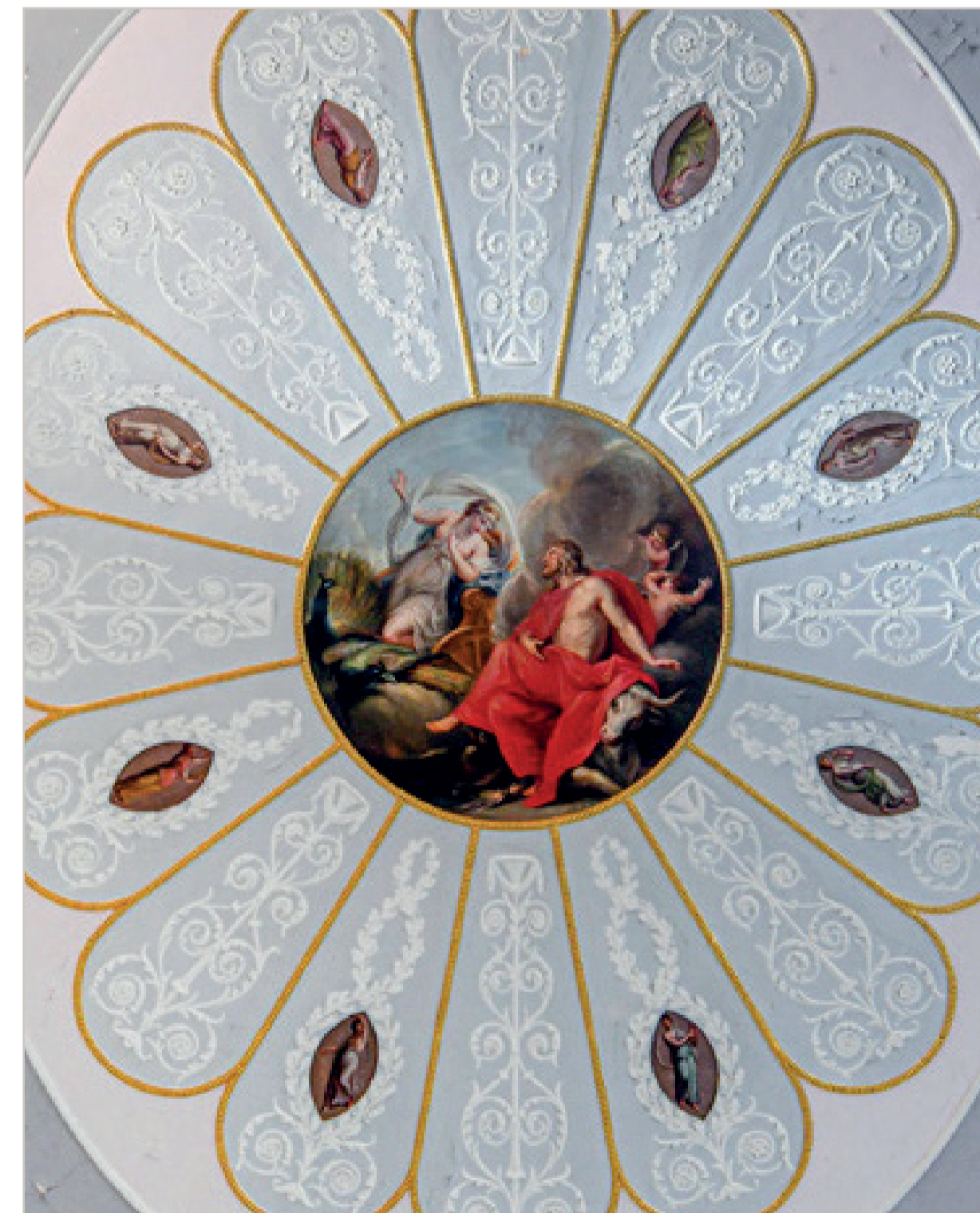
Restoration of the Building and Historic Features
